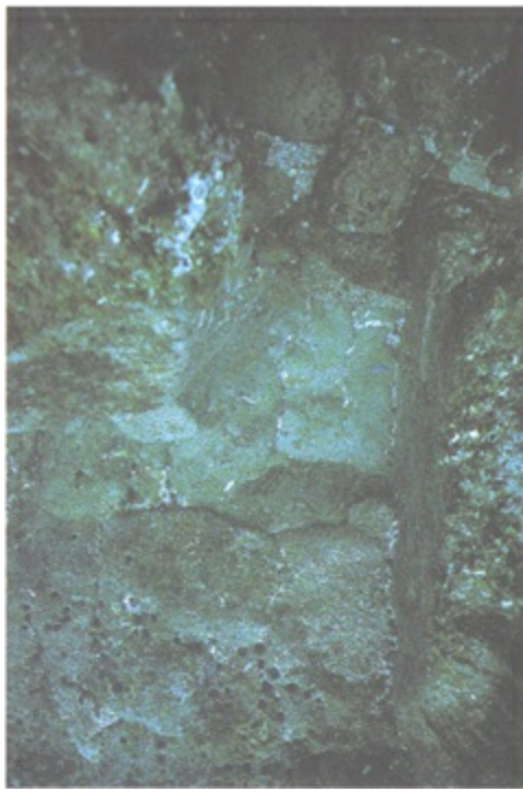
59. Exposed masonry blocks in the Taiwan underwater wall.
